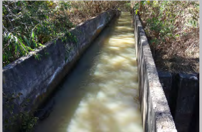
An obstacle that nobody in their 60's should try to overcome— proof supplied by author (photo by Ben Cantrell)
